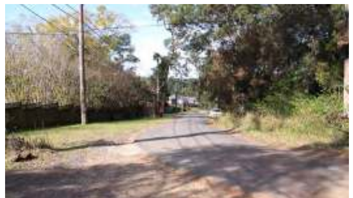
05 View east along Wallana Crescent.
