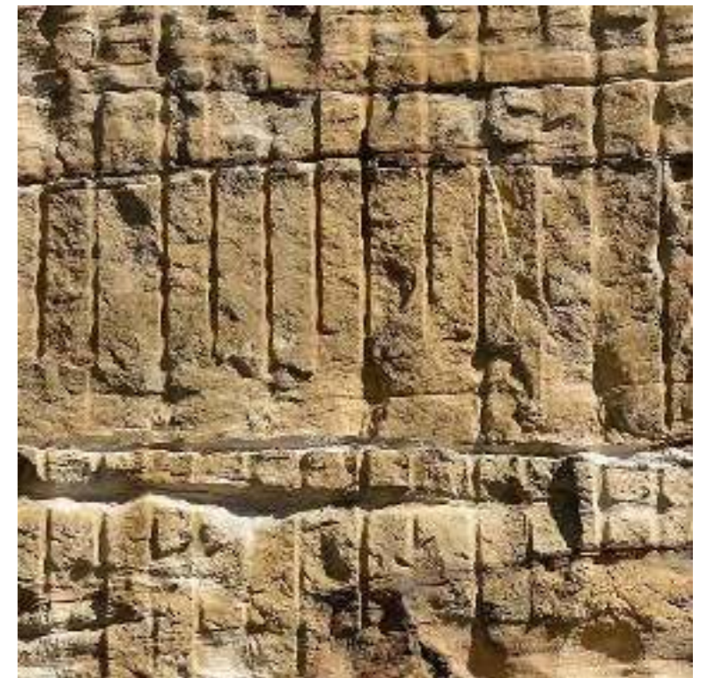
REFERENCE IMAGE: SANDSTONE CUTTING WITH VERTICAL SAW CUTS
