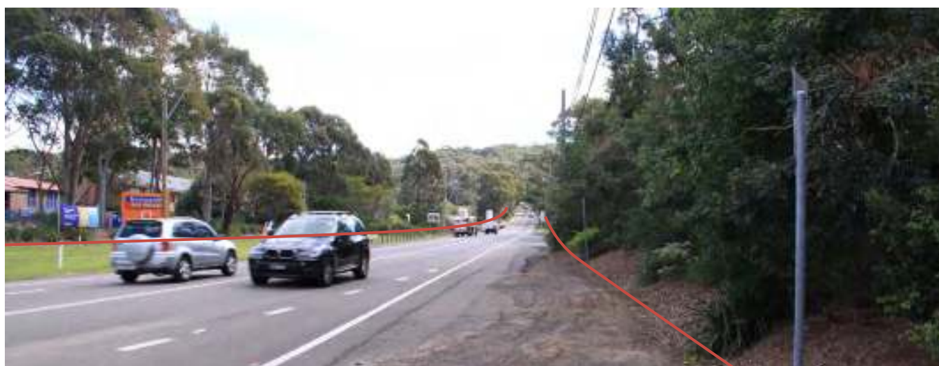
Figure 4.2.22: Existing view looking west along Mona Vale Road on the edge of Landscape Character Zone 8 and towards Landscape Character Zone 6.
