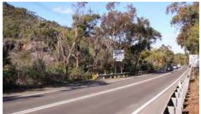
02 View east along Mona Vale Road.
