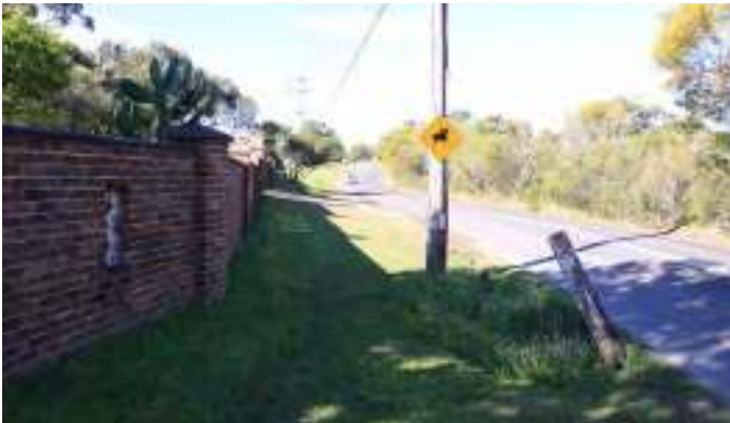
01 View east along Lane Cove Road.
