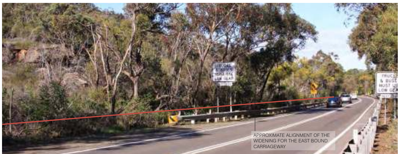
Figure 4.2.5: Existing view looking east along Mona Vale Road from within Landscape Character Zone 3.
