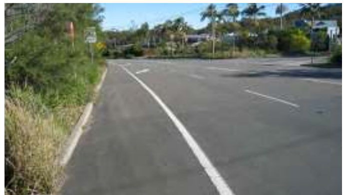
03 View south down Manor Road from close to Mona Vale Road.
