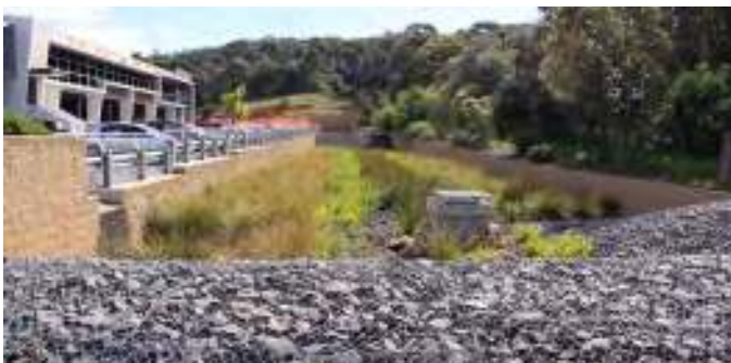
04 View west over the blockwork lined detention basin towards the escarpment.
