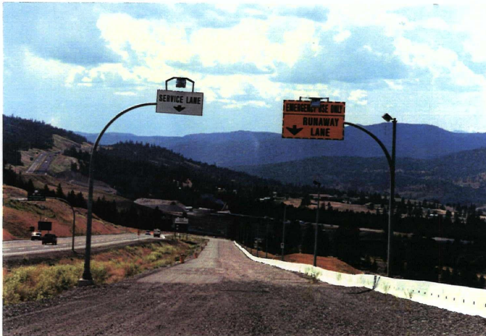
Figure 3.6 Gravel Entrance Lane Prior to the Arrestor Bed, the Arrestor Bed, and the Service Lane
