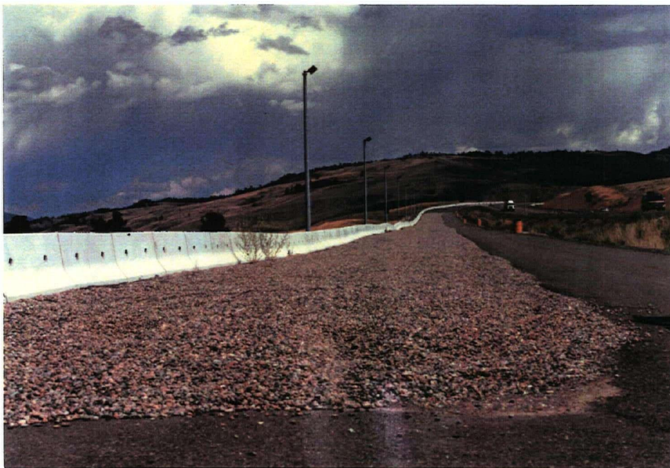
Figure 3.7 End Conditions of the Arrestor Bed
