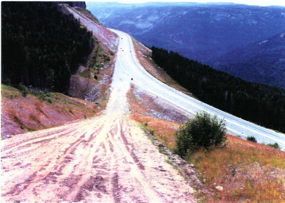
Figure 3.4 Top View of the Ascension Lane and Surface Conditions
