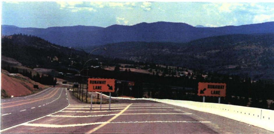
Figure 3.5 Entrance to the Runaway Lane at Hamilton Hill
