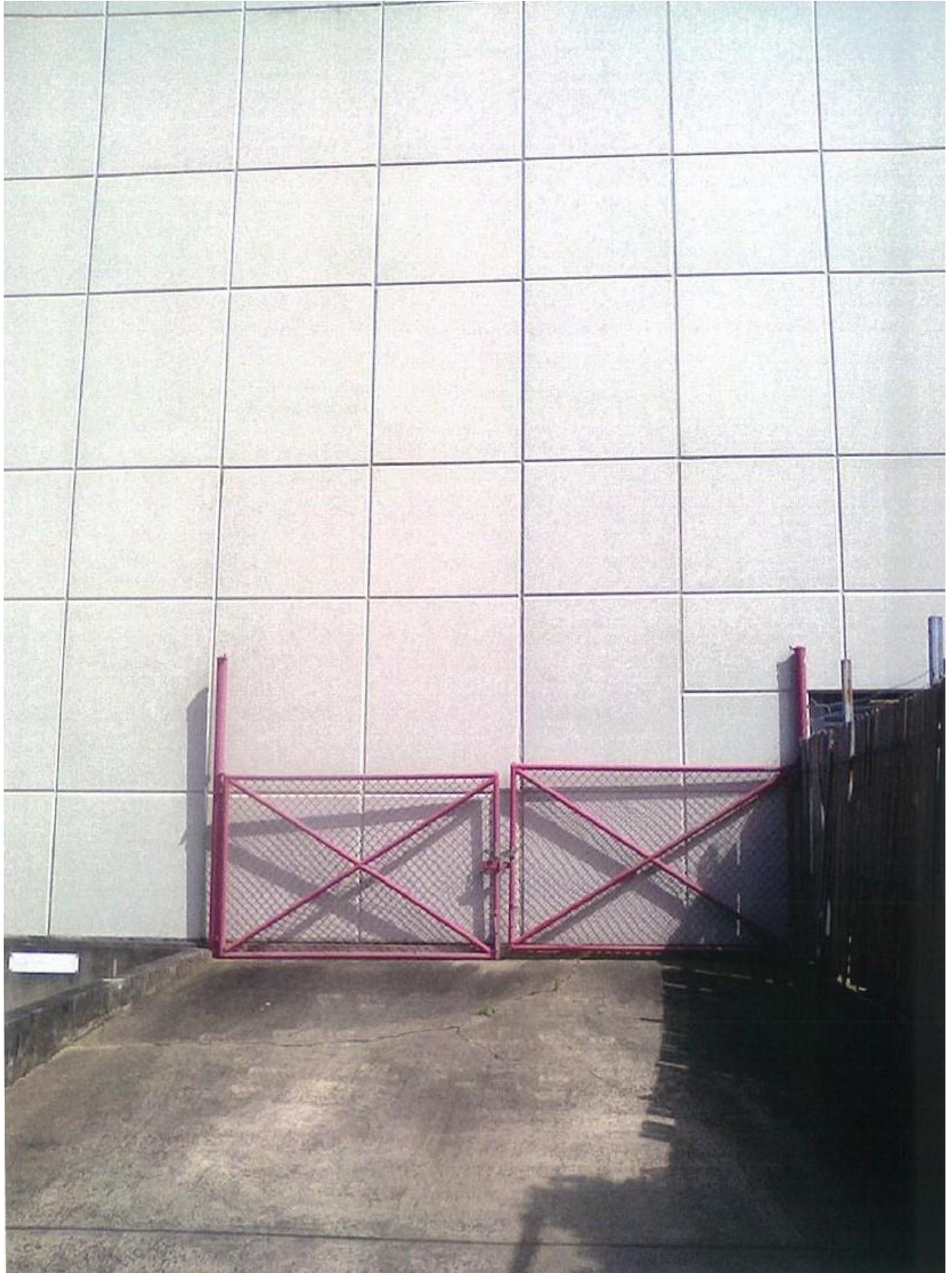
Photo 8: Access – to Post Office from Post Office Car Park
