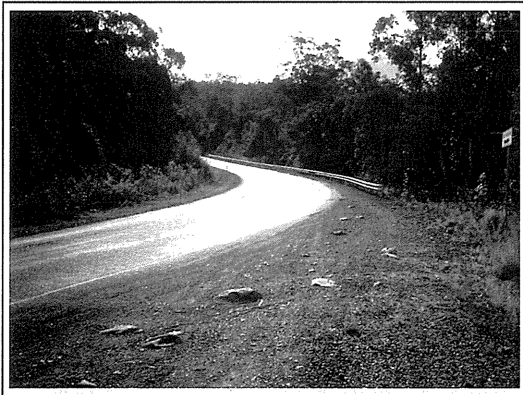
Photograph # 1 – Start of Arrester Bed looking along Thunderbolts Way
