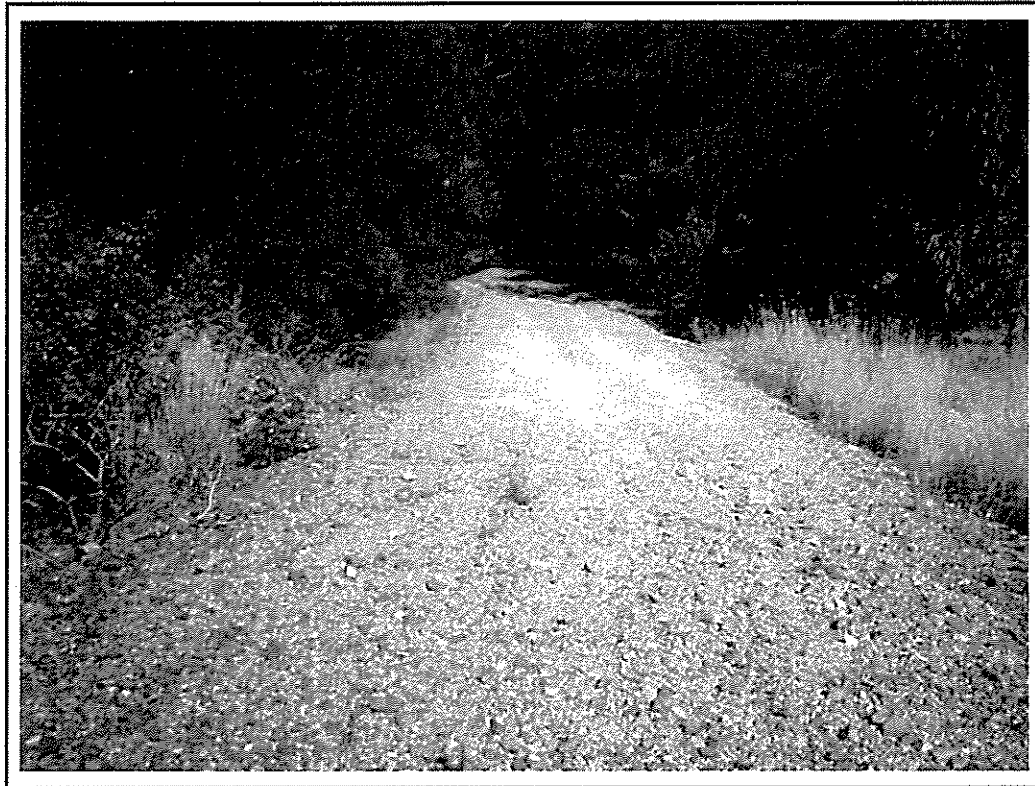
Photograph # 4 – Approximately half way along the Existing Arrester Bed
