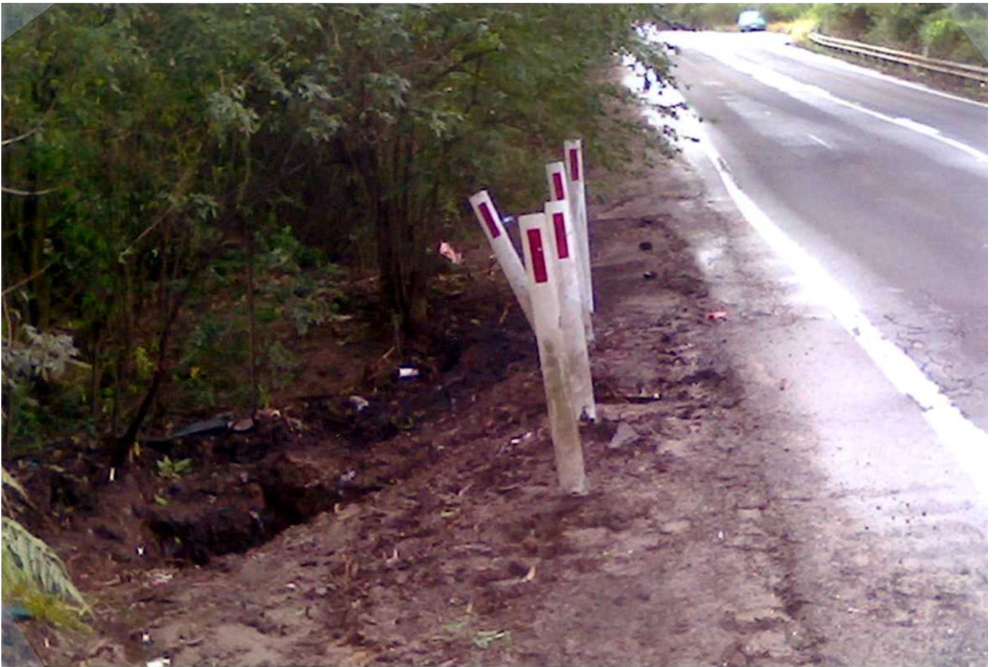
MINIMAL CLEARING OF A PROBLEM DRAIN BY CONNEX-SYDNEY
