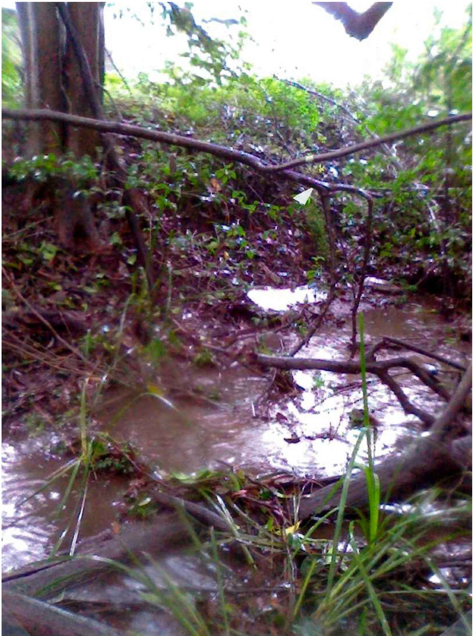
RUNOFF IN SWALE EAST OF BLOCKED DRAIN WITH WATER MOVING EAST TOWARDS WHALE ROCK
