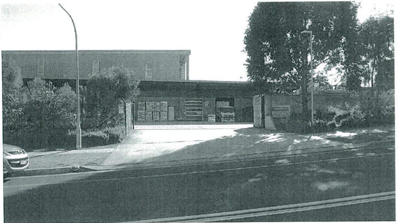
Photograph 2: Entrance to premises from Jubilee Avenue
