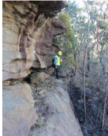
Figure 3-2: Geotechnical constraints to the south of the existing alignment, east of Kimbriki Road.
